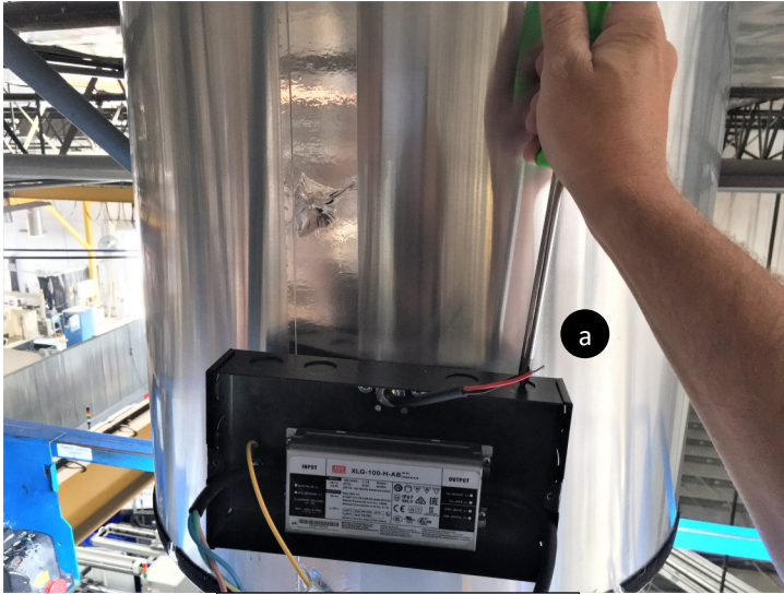
Remove knockout for control wires
