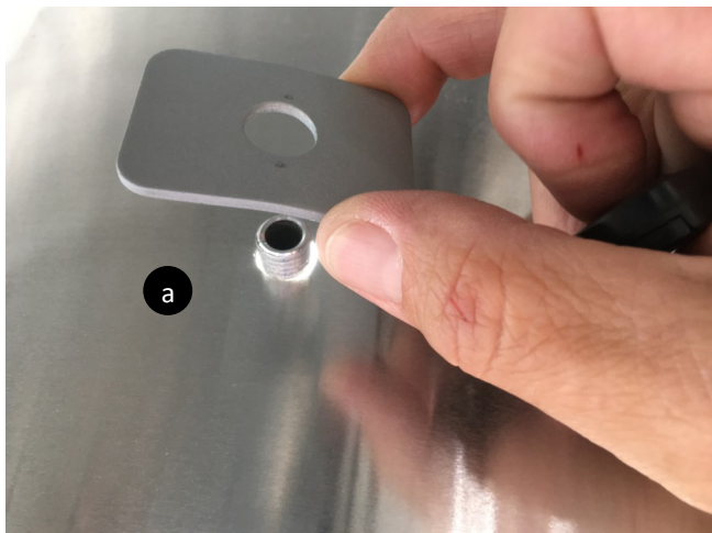
Place metal washer over LED fixture threads on outside of tube.
