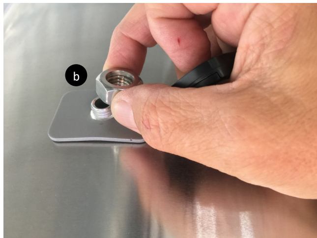
Secure LED fixture with nut.
