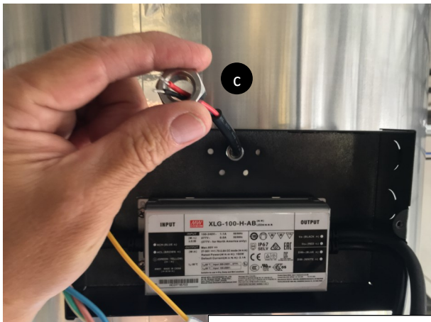
Install nut over threads and tighten to secure with wrench.
