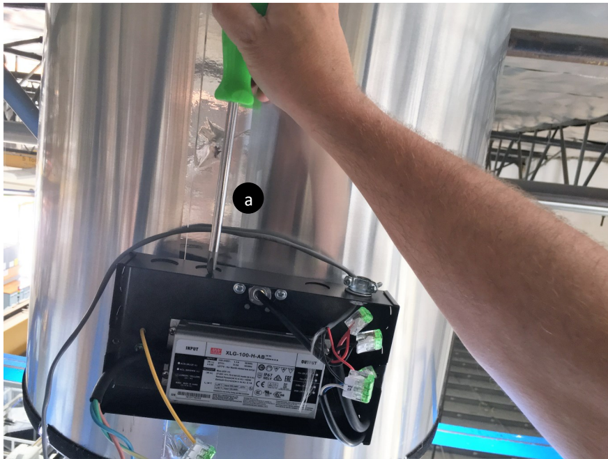
Remove knockout for control wires
