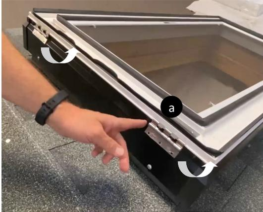
Screen can be flipped for access to plunger pins from interior or from roof.
