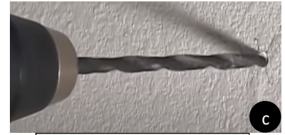
Drill marked fastener locations
