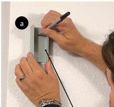
Mark fastener holes onto wall
