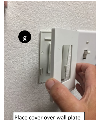
Place cover over wall plate
