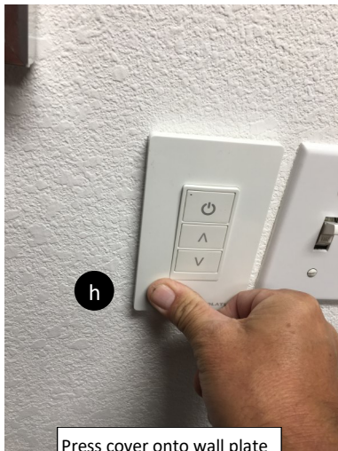
Press cover onto wall plate until it snaps into place
