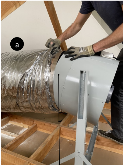
Pull ducting evenly over fan transition.
