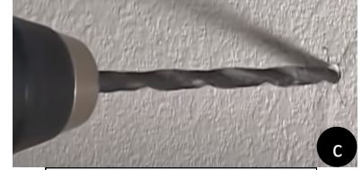
Drill marked fastener locations
