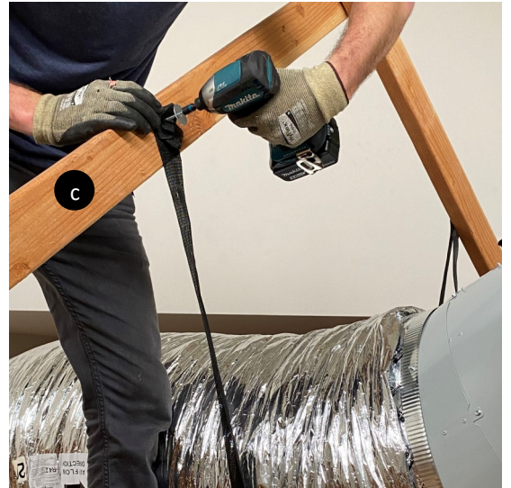
Use a custom length of strapping material to install a center strap on the ducting to keep the ducting in an optimum curve and maximizing air flow. Fasten each side of strapping with 1-1/2 in. Hex Head Drill Tip Screws and Washers.
