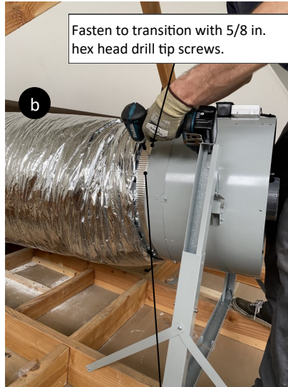
For best results, apply foil tape over duct and collar connection.
