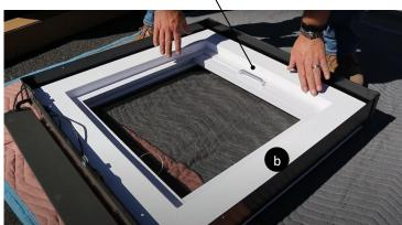
Ensure screw fastener is installed straight.
