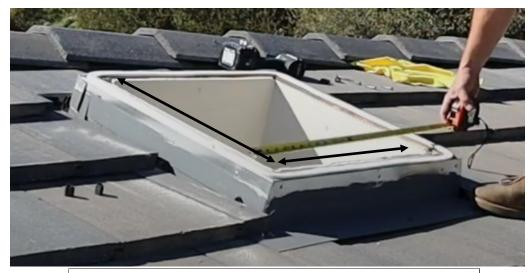
Measure inside dimension of skylight chase to determine if the curb will need to be raised. In the example below, the skylight being installed is a SL2828.
