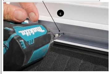
Fasten shade to operable base with four (4) provided screws
