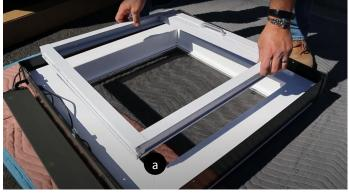
For best operation, ensure shade handle is installed on the upslope
