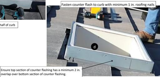
The skylight is ready for installation. To install skylight please refer to Solatube HSE Skylight Installation Instructions (P/N: 952620) at www.solatube.com
