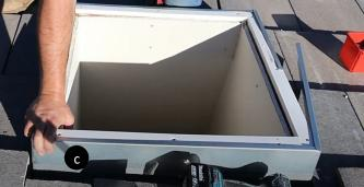
Form counter flashing snug around top half of curb
