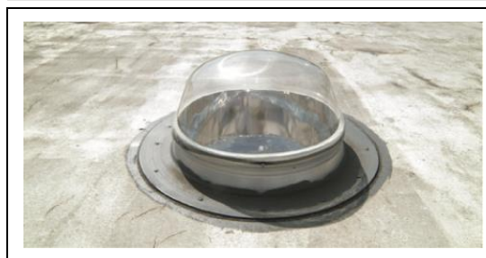
Figure 4 Flat roof flashing installation
