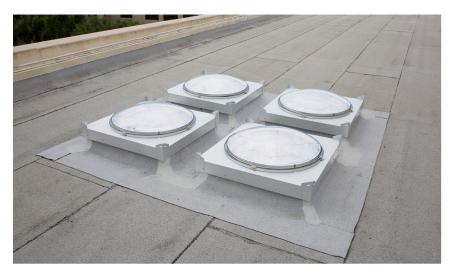
The unique installation included four (4) SkyVault M74 with Amplifier units, bundled together with a custom diffuser to provide maximum daylight. The installation was further customized with the installation of LEDs for both daylighting and night use.
