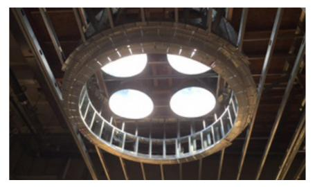
"Bringing in daylight to a two-story lobby was no small feat," according to Angela Chiang, LEED AP, Project Designer at LPA, Inc. "We chose a unique configuration of four SkyVault units with Amplifiers installed as a group in one large nine-foot diameter lightwell."
