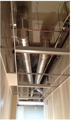
Typical commercial installations have tube runs of four to five feet. This project required horizontal tube runs of 17 feet, with minimal light loss.
