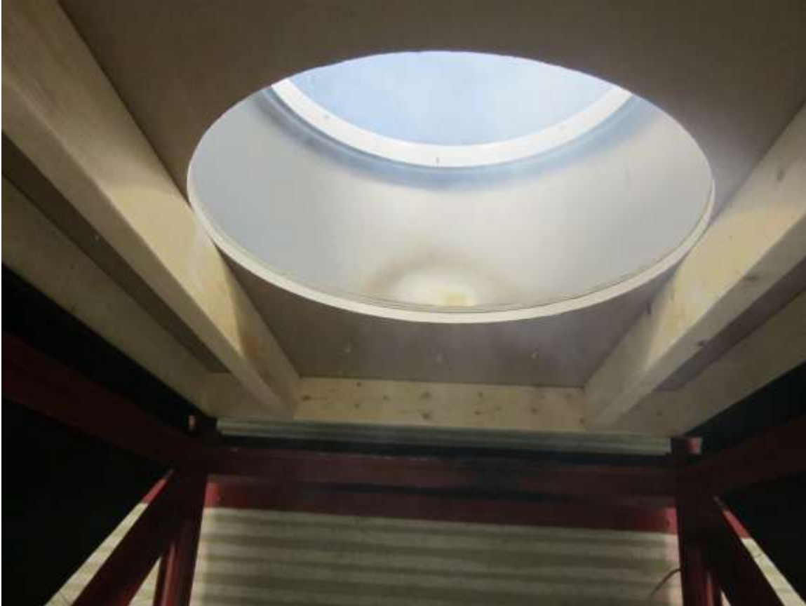
Photo No. 4 Inside of 330 DS Flashing at Test Conclusion
