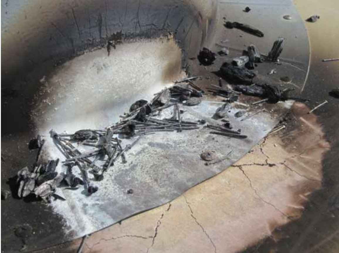
Photo No. 9 Warping of 750 DS Flashing
