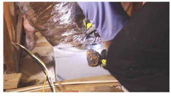
Place Ducting onto Damper Box Ensure the duct air flow arrow is pointed towards the fan.
